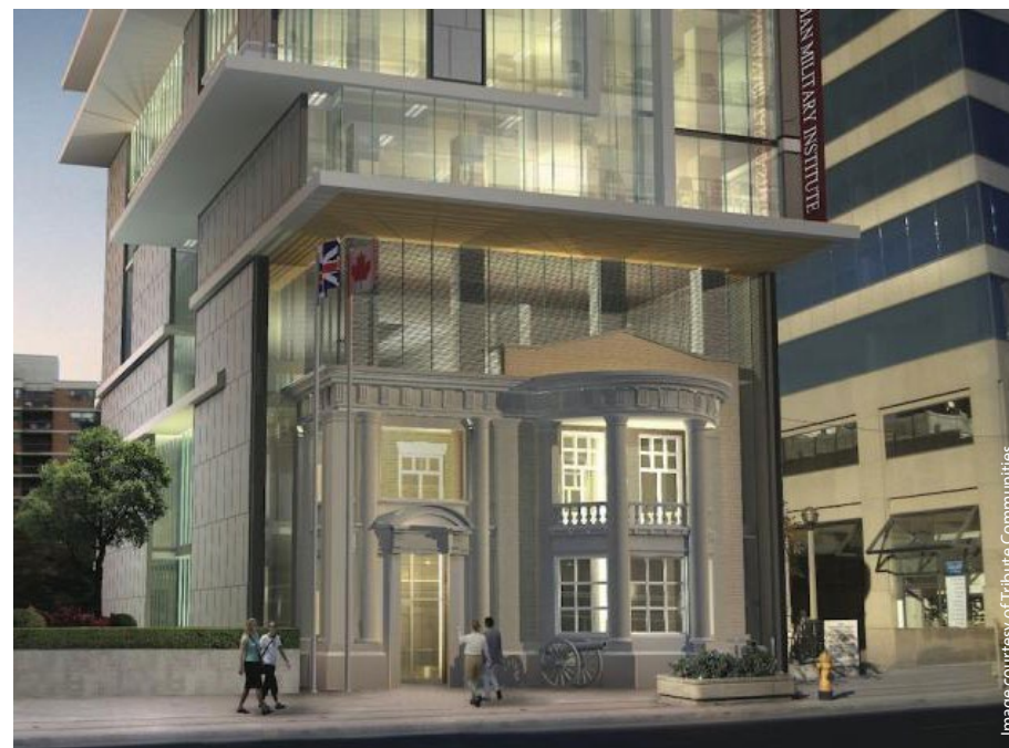
The parking-free Tribute Communities high-rise building on University Avenue is well connected to street level without parking ramps.
